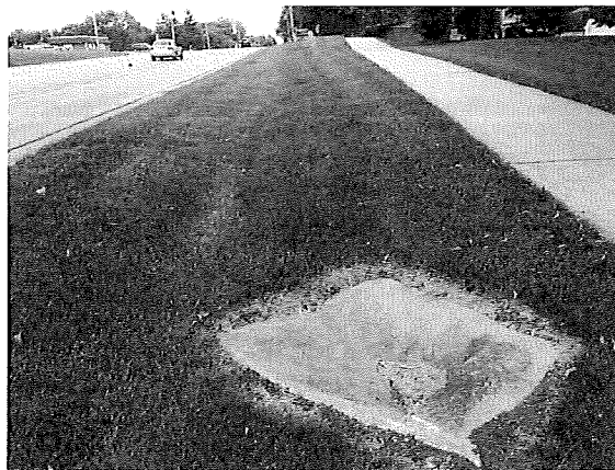
Figure 4. Grand Avenue southside swale inlet
