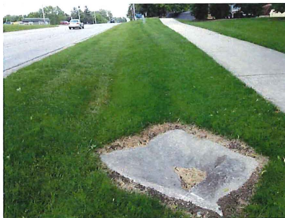
Figure 4. Grand Avenue southside swale inlet
