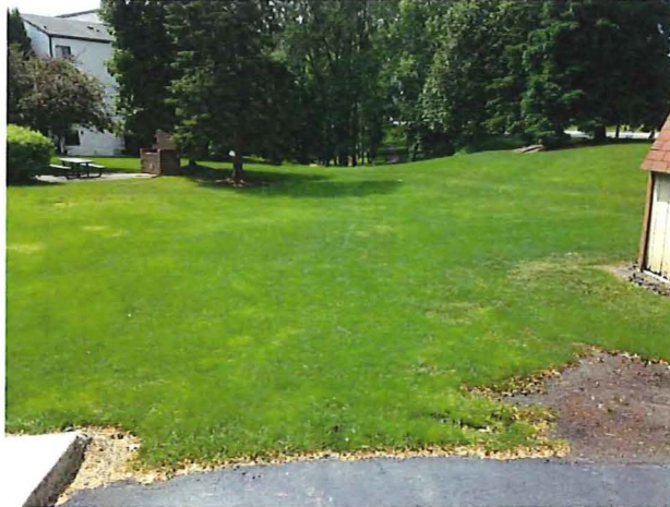
Figure 7. Grass swale off south corner of east side parking lot
