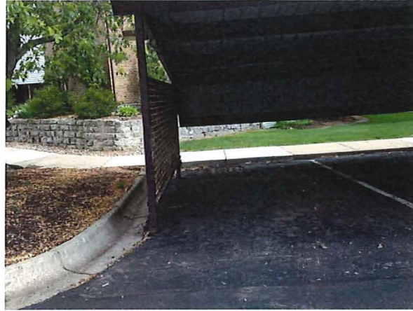
Figure 5. East side Parking Lot Inlet (to pond)
