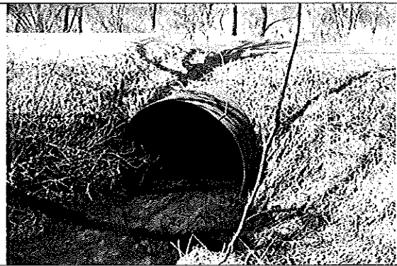
Existing inlet in relation to the roadway
