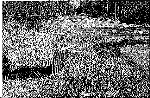
Existing outlet relative to the clear zone
