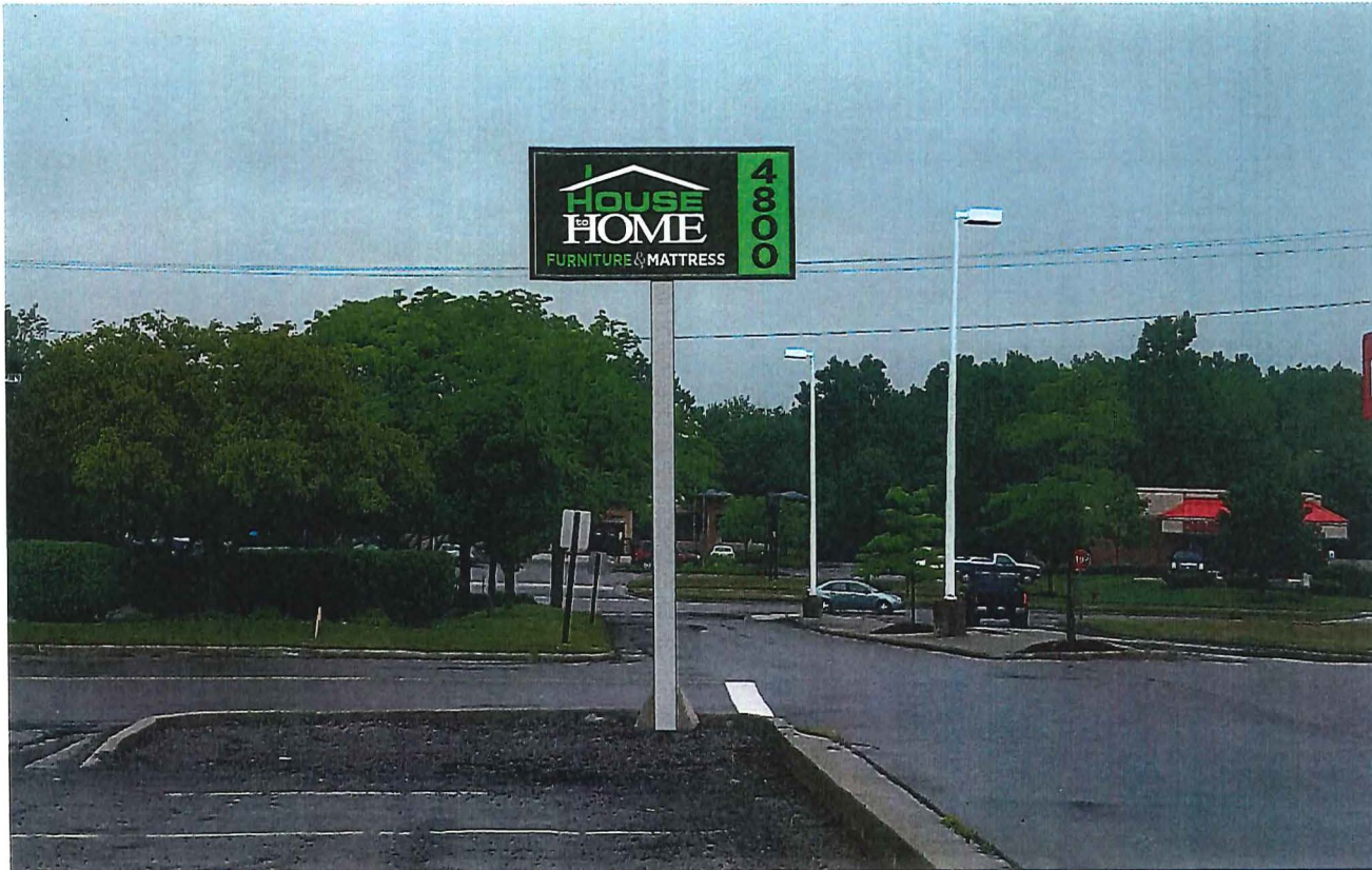
PYLON SIGN 4' x 8' Cabinet (moved from former location) Illuminated painted aluminum sign cabinet, new faces 3sqft address "4800" 16' high painted steel pole
