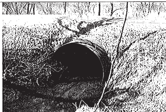
Existing inlet in relation to the roadway
