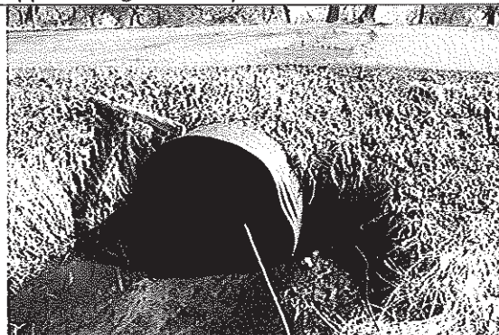
Existing outlet in relation to the roadway
