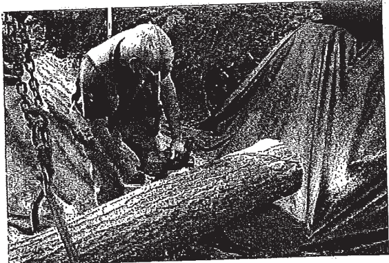
Construction of the Log Stilling Basins was completed onsite to ensure flush angles for durability.
