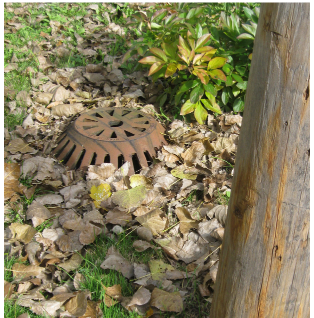
Figure 14. Catch-basin #16 on Columbia Street.
