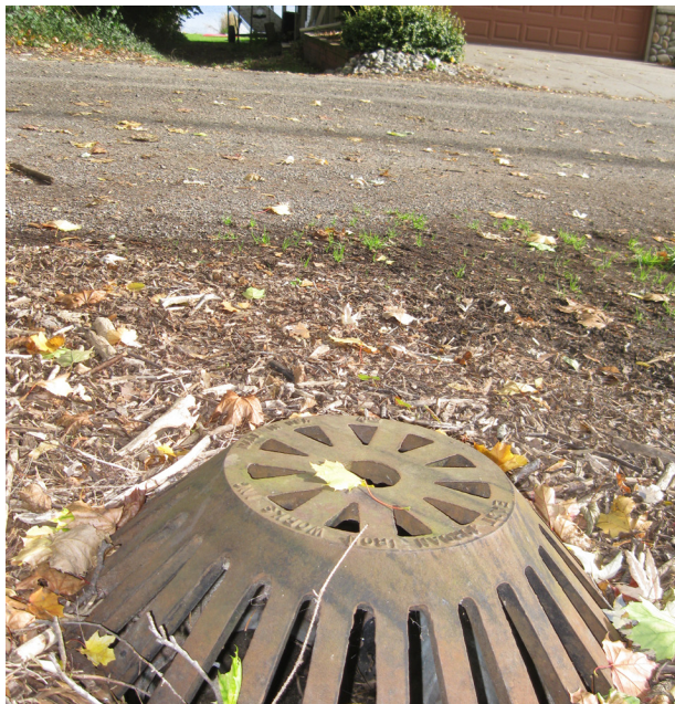
Figure 13. Catch-basin #15 on Columbia Street.
