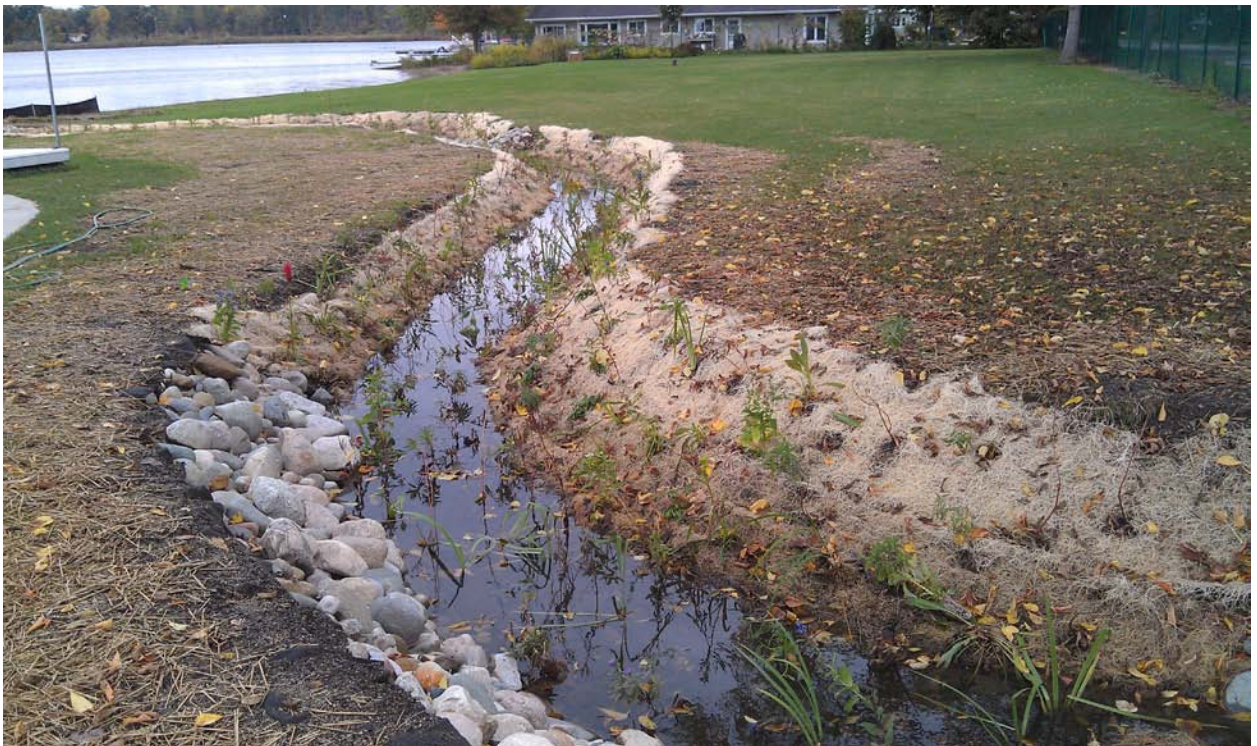
Figure 12. Lake Lansing Park South installed bioswale.
