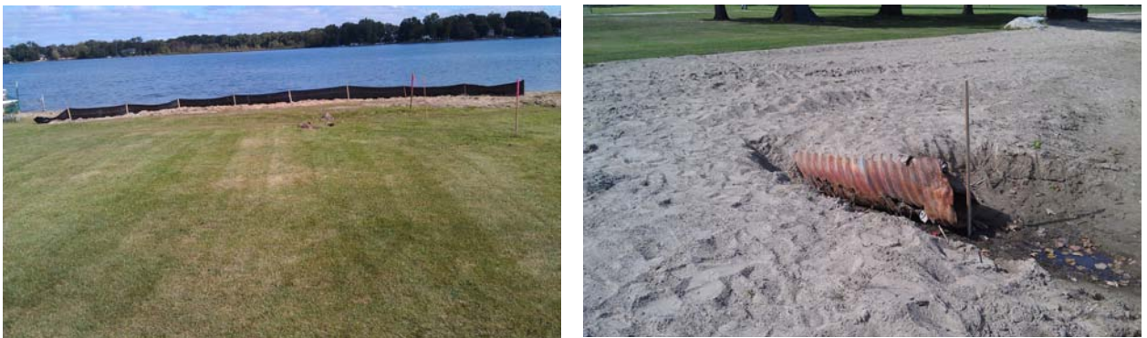
Figure 11. Lake Lansing Park South area before bioswale construction.
