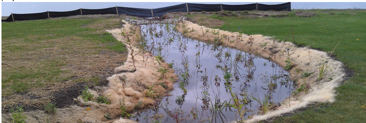
Figure 1. Installed bioswale at Lake Lansing Park South.
