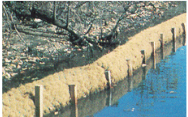
Figure 14. Coir logs for erosion control.
