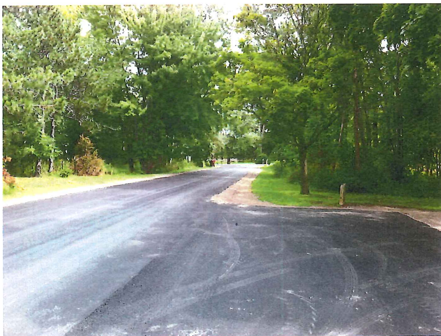
LEGG PARK – entry and small parking area has been paved
