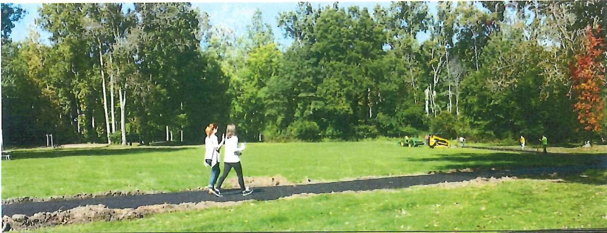
WONCH PARK – paving was completed on September 22, 2014. Restoration is in progress.
