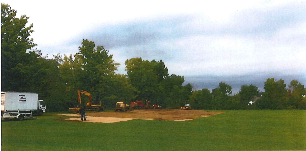
NEWTON ROAD PARK – entry and parking area under construction
