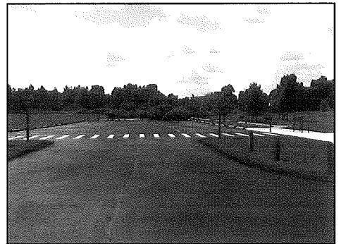
Parking Lot Resurfacing—N. Meridian Rd. Pk.
