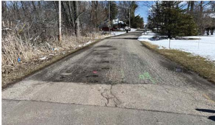
Figure 1 – Roadway in the vicinity of B-5
