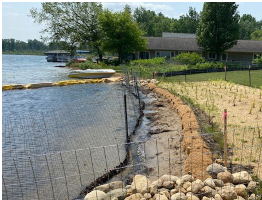
Natural shoreline restoration demonstration project currently being installed at the south end of the Lake Lansing Park South county park.
