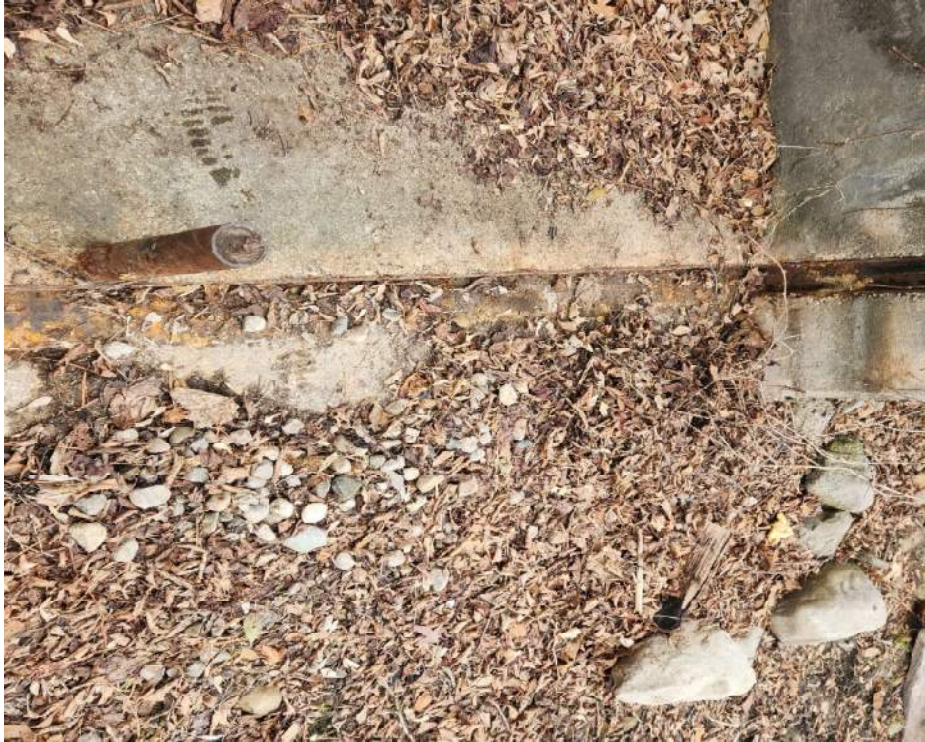
Figure 15 – Stop Log Channel
