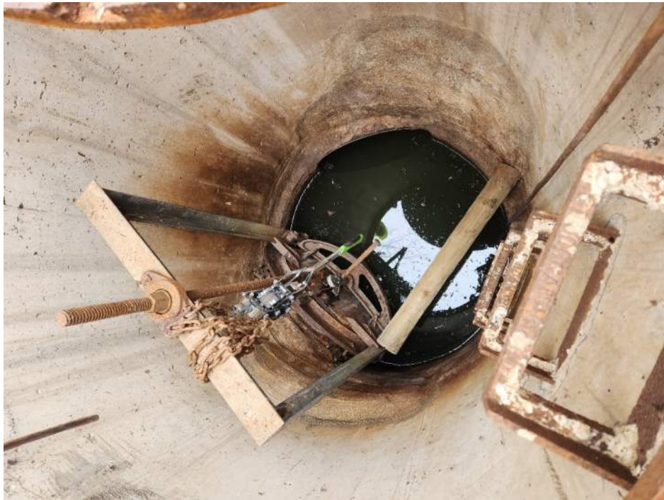
Figure 2 – Slide Gate (Valve)
