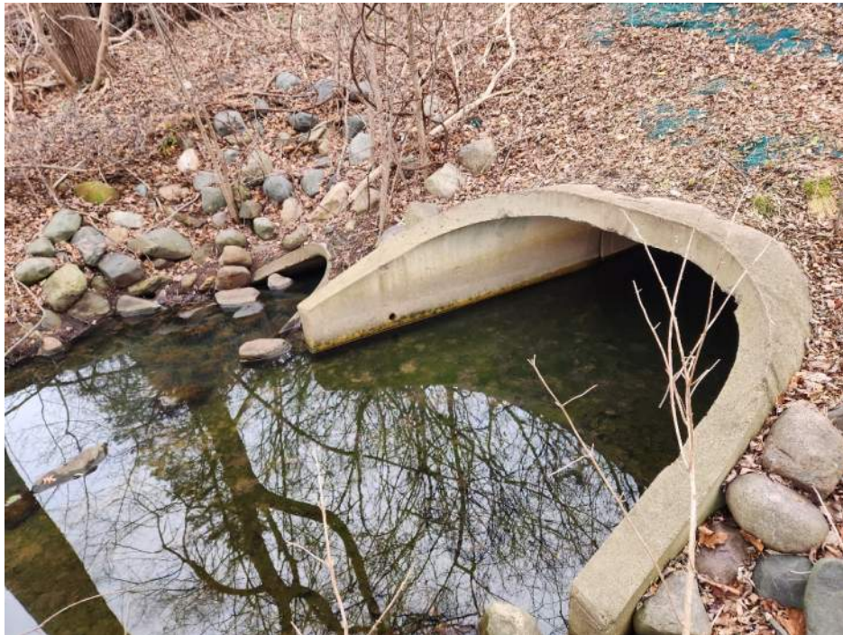
Figure 14 – Marsh Rd. Outlet Structure: West End
