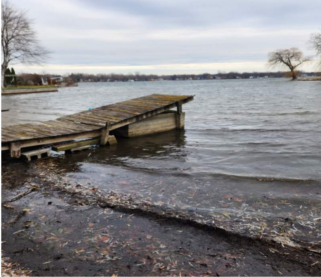
Figure 17 – Dock Condition over the inlet structure
