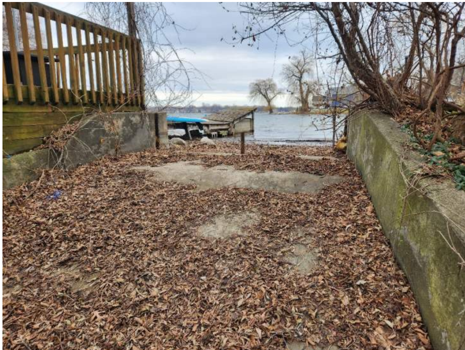
Figure 10 – Spillway looking towards the Lake
