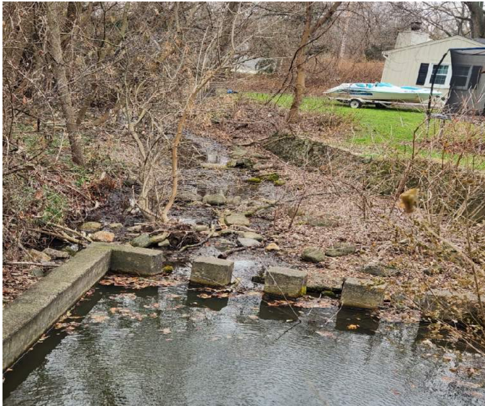
Figure 12 – Open Channel Looking downstream
