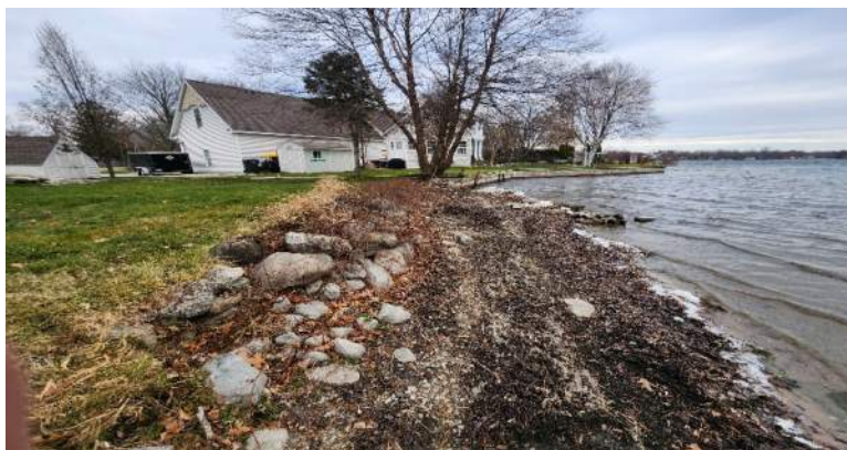
Figure 18 – Seawall right of Spillway
