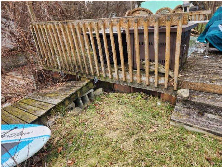
Figure 8 – Sheet Piling Right of Spillway
