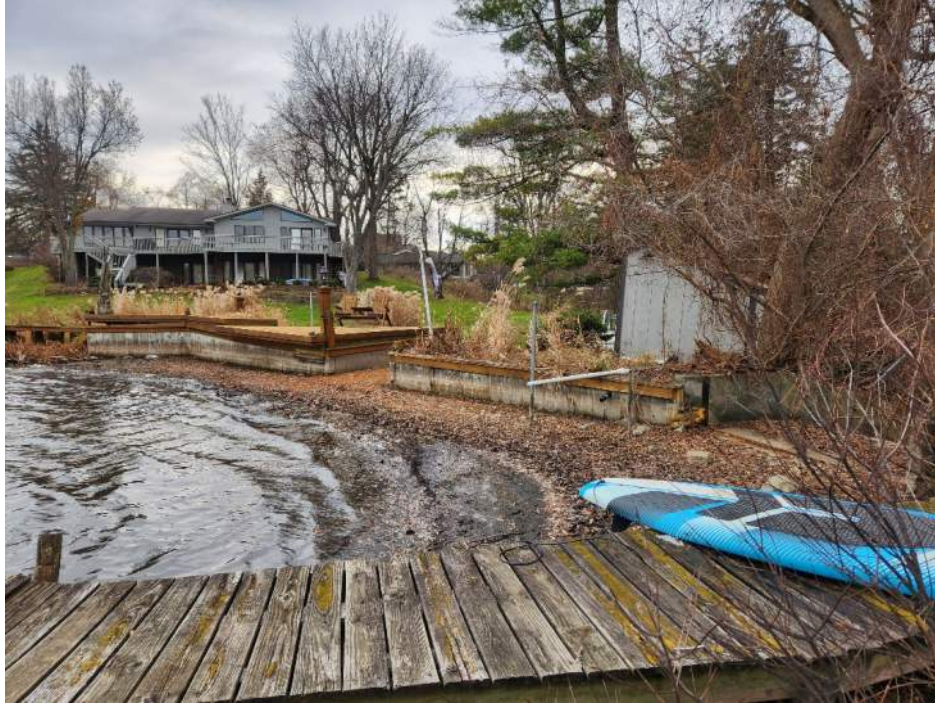
Figure 5 – Sea Wall and Approach to Spillway from the Dock location
