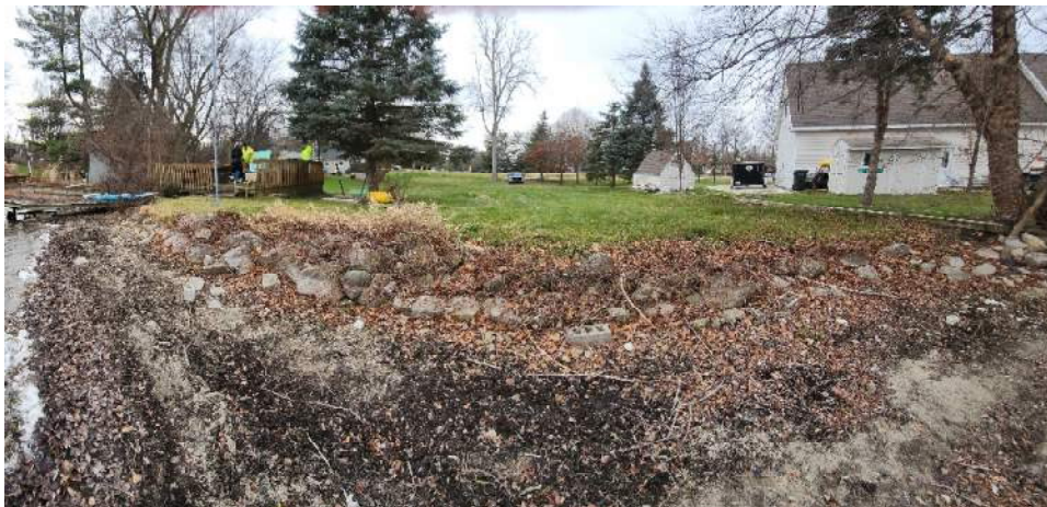
Figure 6 – Riprap Shoreline Right of Spillway from the Dock location
