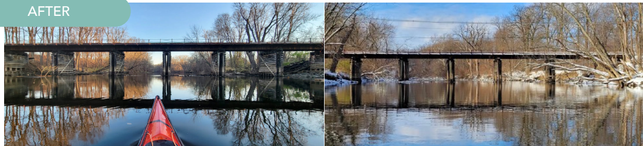
GRAND RIVER RAILROAD BRIDGE
