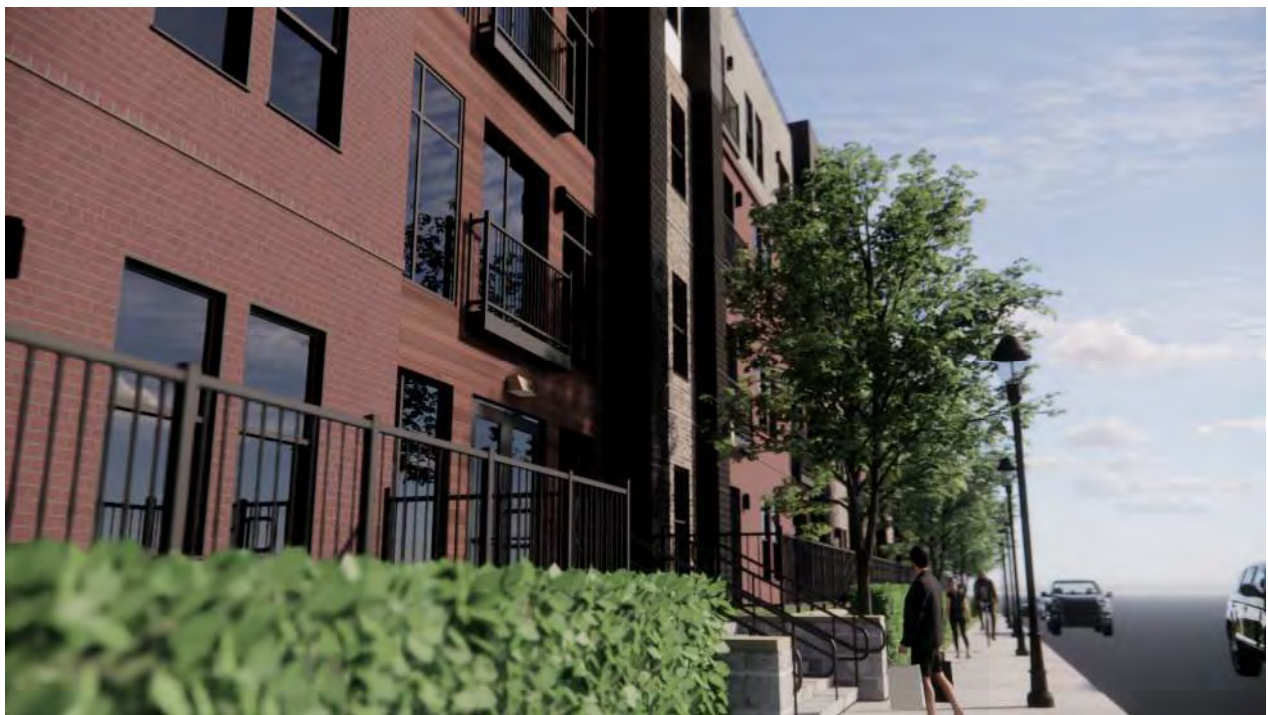
Block 2 – Street View (looking North along Okemos Road)
