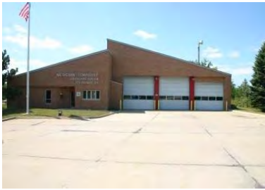
Station 93 - Engine, Ladder, Ambulance, Rescue Water, Safety Trailer, District 1 Mass Casualty Trailer, "Jaws of Life"
