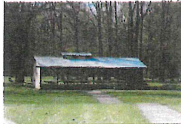
Wonch Park - pavilion (no electricity) and restroom building - capacity 30-50
