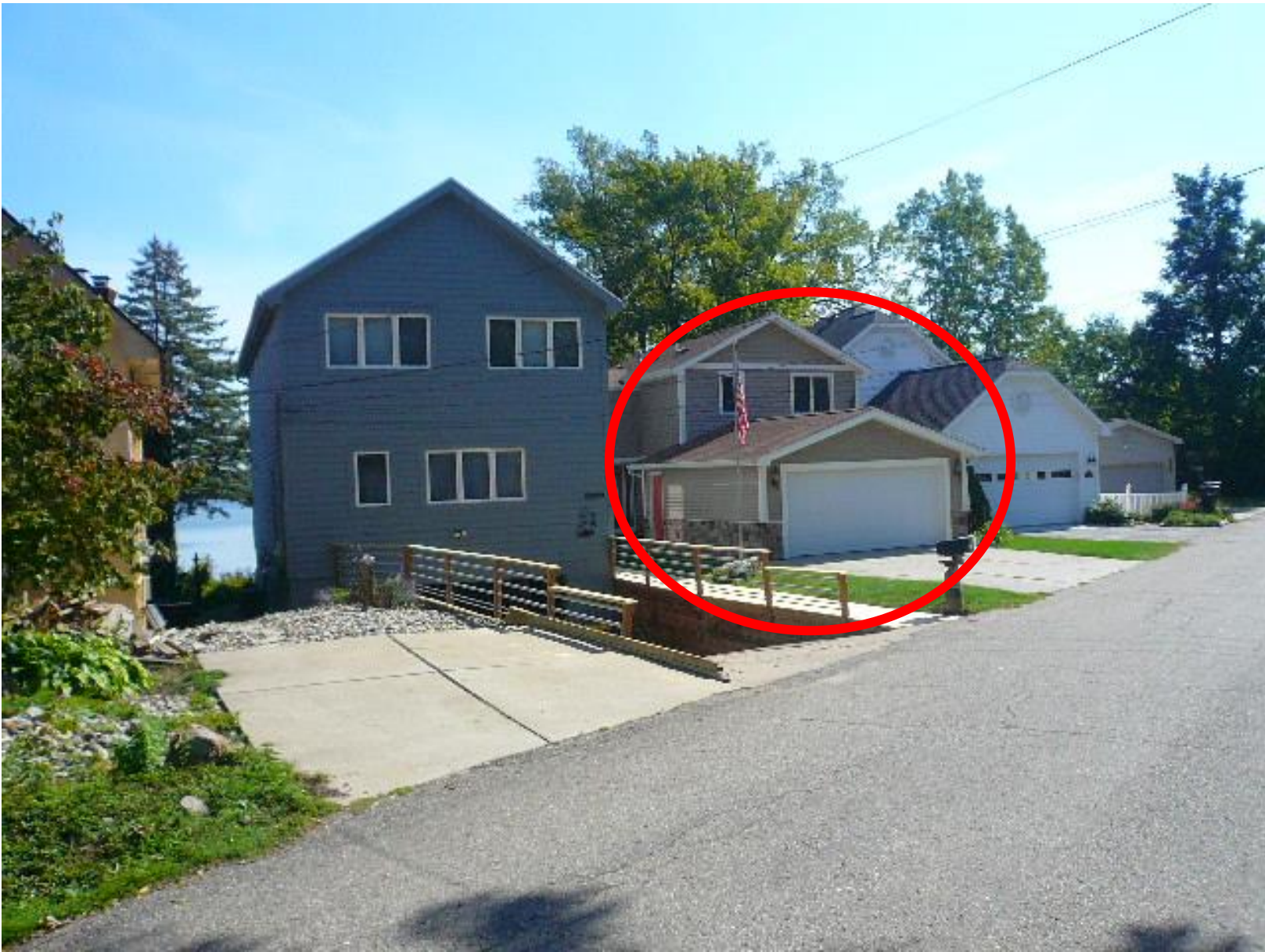
Photo showing street view of house to the north
