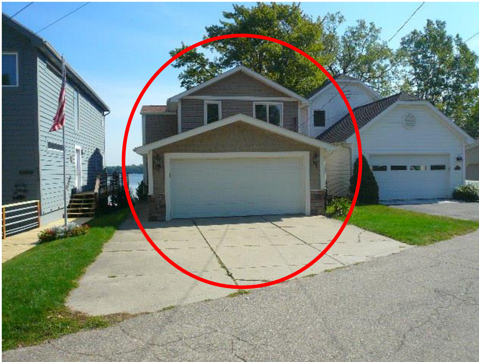
Photo showing existing garage and drive at 6074 Columbia
