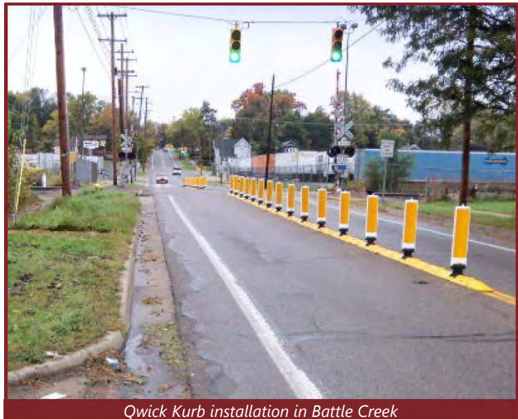
Qwick Kurb installation in Battle Creek
