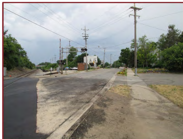
Haslett Road (CN RR) Driveway in NW Quad inside of gate arm
