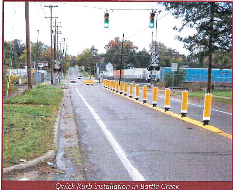
Qwick Kurb installation in Battle Creek
