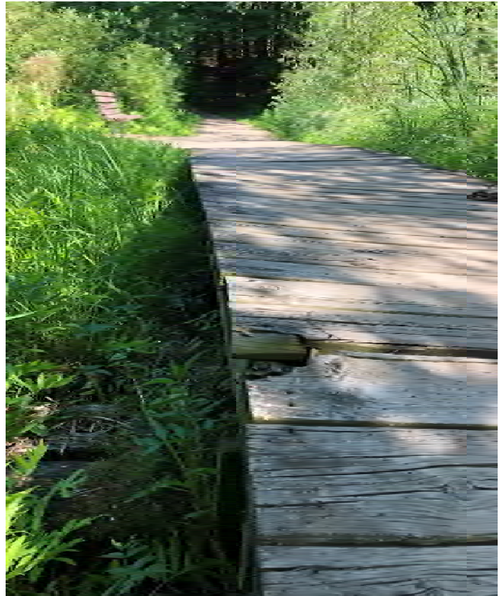
Above Left: Missing and heaved boardwalk planks are a safety hazard. Above Right: Deteriorated boardwalk planks. There are no existing curbs or bumpers on the boardwalk, causing a potential roll-off hazard for wheelchair users. Below: Deteriorated entrance sign.
