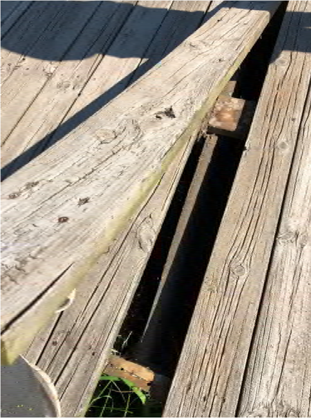
Above Left: Missing and heaved boardwalk planks are a safety hazard. Above Right: Deteriorated boardwalk planks. There are no existing curbs or bumpers on the boardwalk, causing a potential roll-off hazard for wheelchair users. Below: Deteriorated entrance sign.
