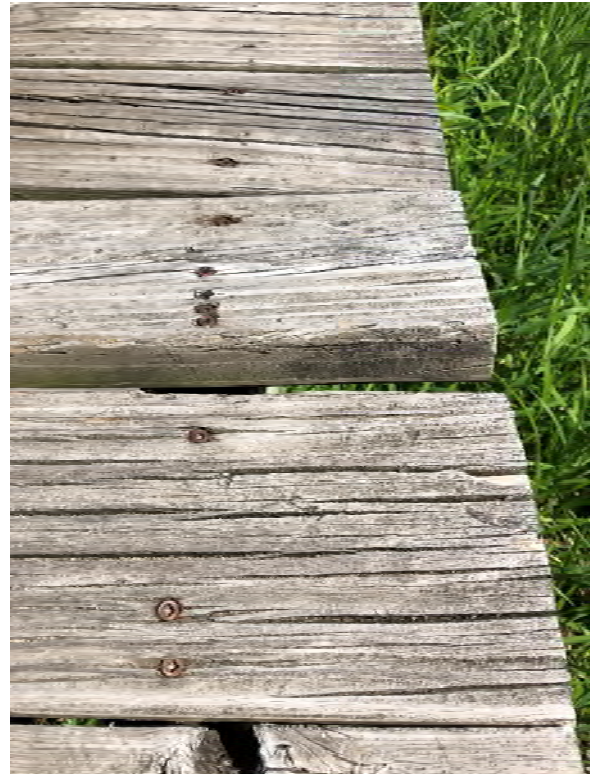
Above right and immediate left: Typical condition of boardwalk planks – deteriorated and heaved, with gaps that are a trip and fall/safety concern.
