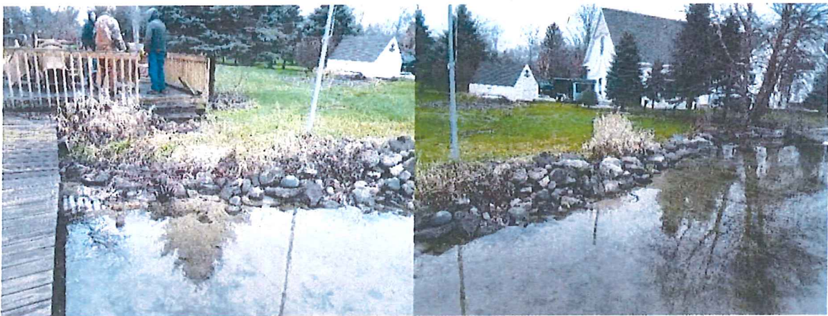
Figure 12 – Riprap Shoreline Right of Spillway
