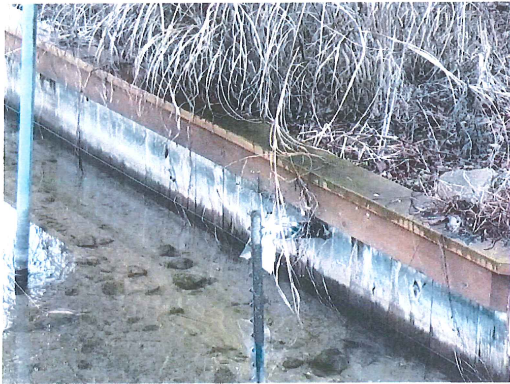
Figure 11 – Concrete Sea Wall Left of Spillway
