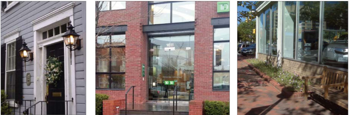
Left to right: Door with TRANSOM; Multi-paned SHOPFRONT windows and glass doors; SHOPFRONT window
