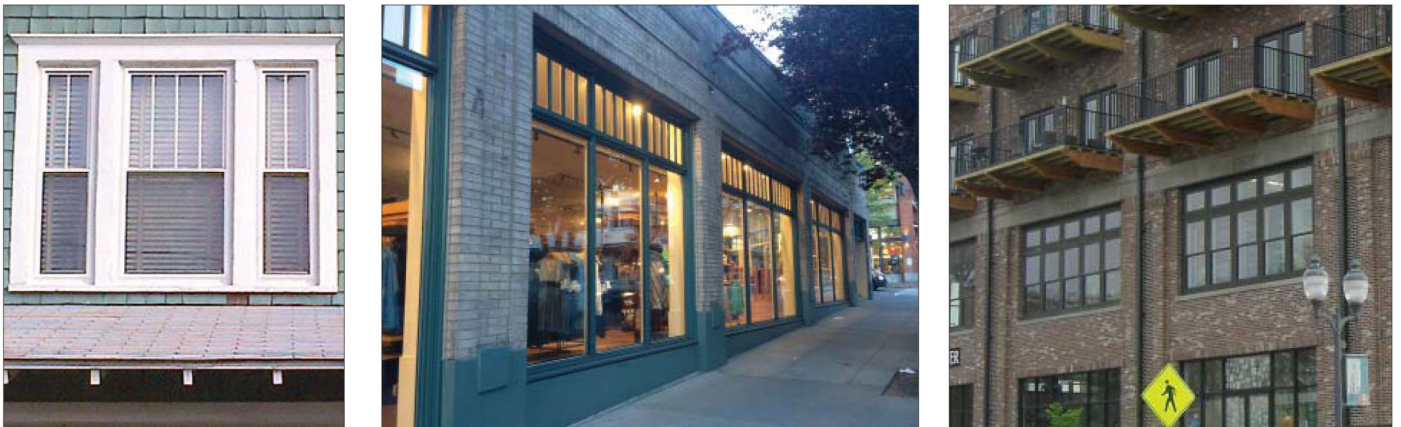
Left to right: Grouped windows; SHOPFRONT frontage; Grouped windows
