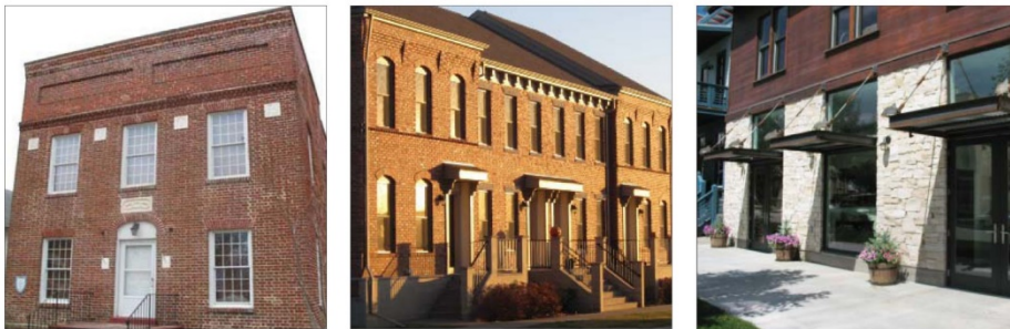
Left to right: Brick building walls; Newly constructed brick townhouses with architectural detailing; Building FAÇADES with limestone ground floor and wood siding above.
