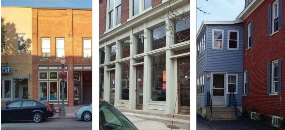
Left to right: Buildings with brick FAÇADE; Cast iron SHOPFRONT with brick second STORY; Material change in a logical location
