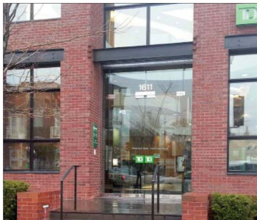
Left to right: Door with TRANSOM; Multi-paned SHOPFRONT windows and glass doors; SHOPFRONT window
