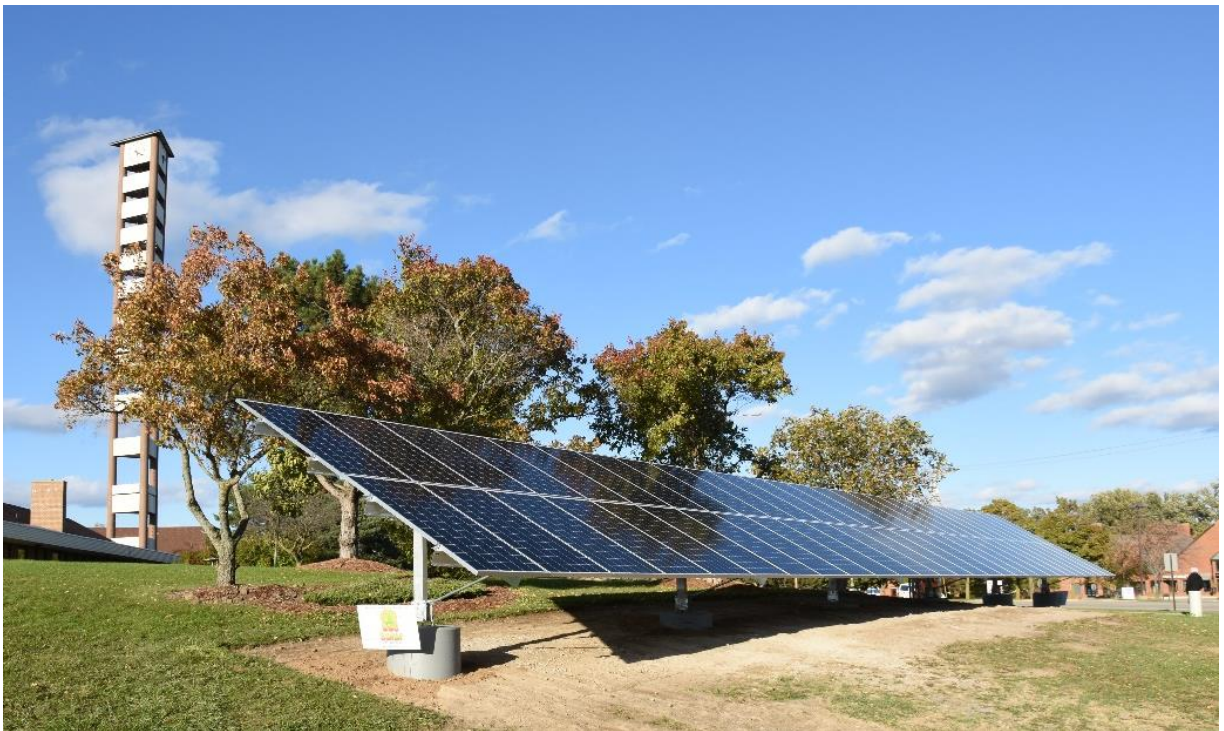
Photo of Meridian's new 20 kilowatt photovoltaic array by Roger Eberhardt, Meridian Energy Team
