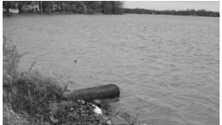
Figure 17. Lake Lansing storm drain outfall.
