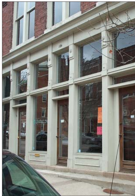
Cast iron shopfront with brick second story
