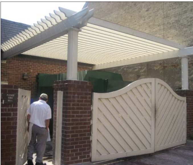
STREET WALL with gates shielding service area
