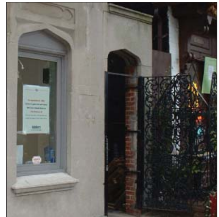
STREET WALL with gate between FAÇADES
