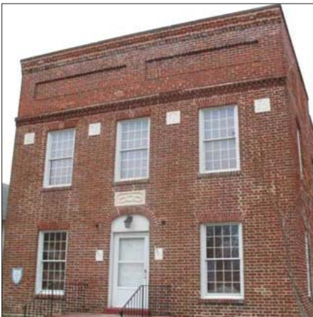
Brick building walls
