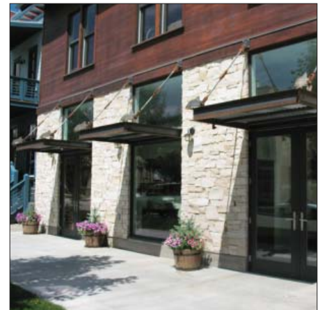
Building FAÇADES with limestone ground floor and wood siding above.
