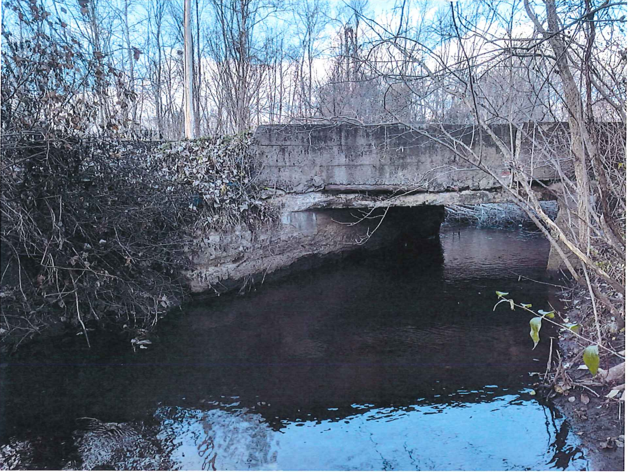
7-1: South of bridge, looking north.
