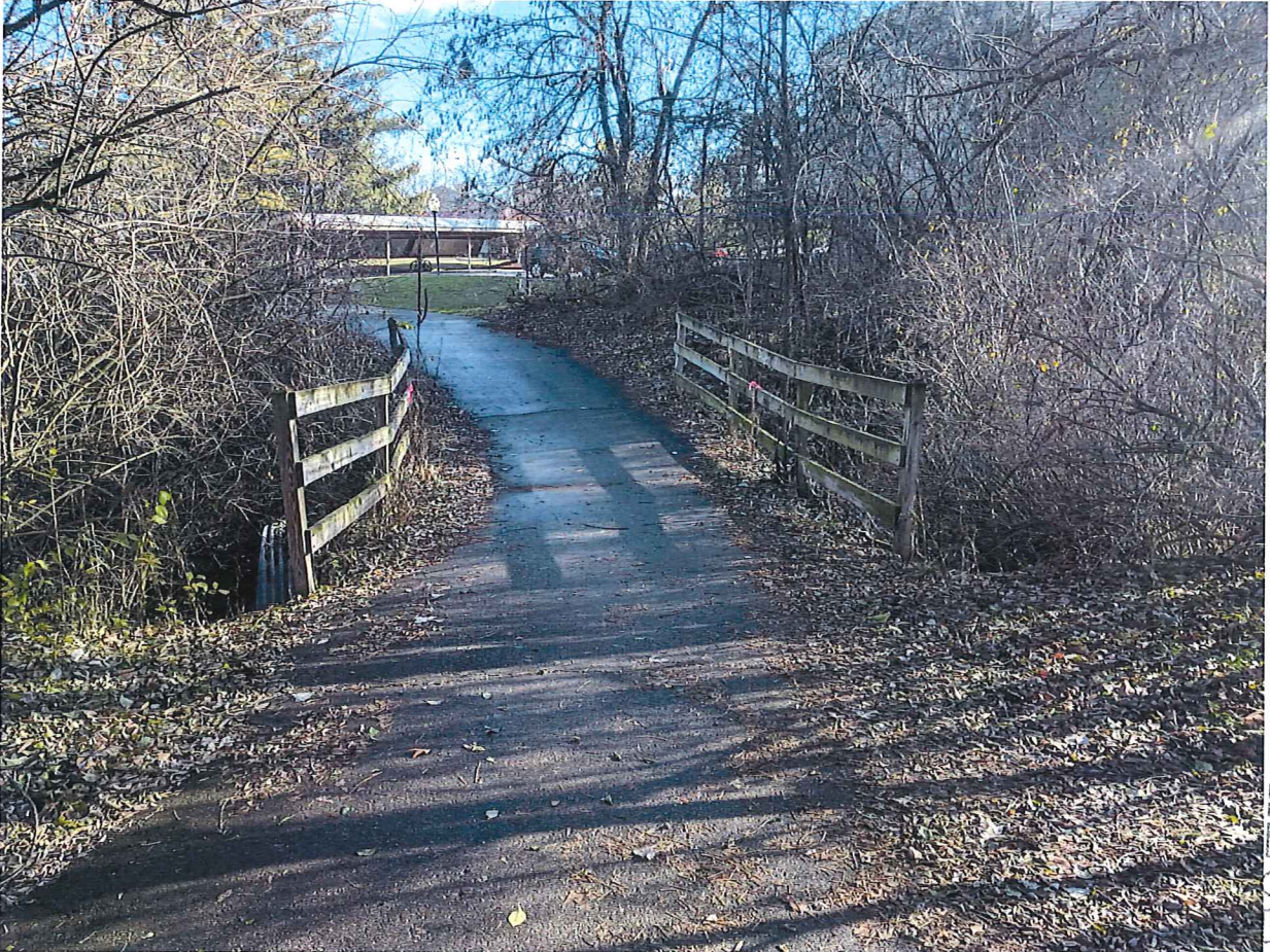
5-2: West of culvert, looking east.
