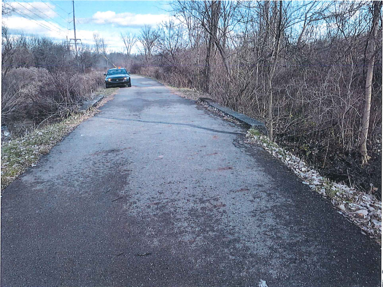
7-2: West of bridge, looking east.
