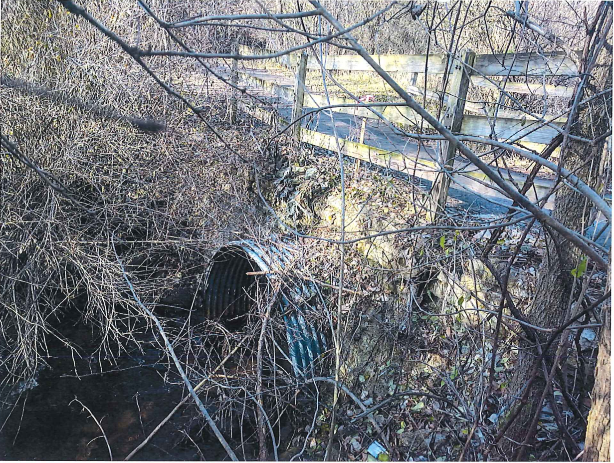
5-1: Southeast of culvert, looking northwest.
