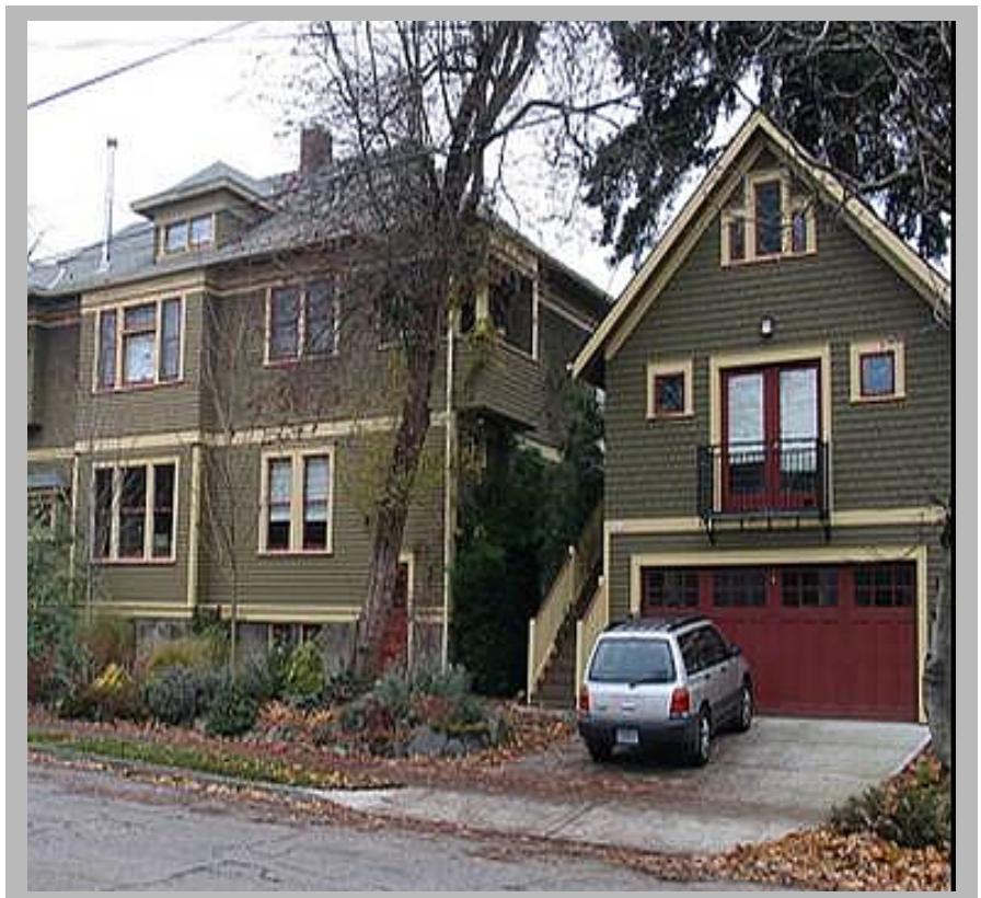
Photo by radworld (creative commons)
