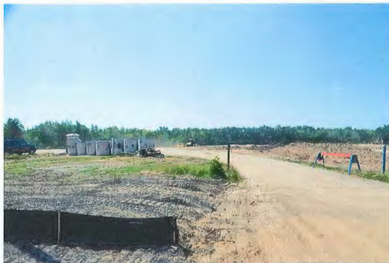
Towner Road Park Construction
