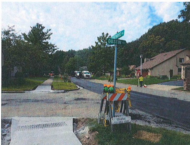
Local Roads Construction
